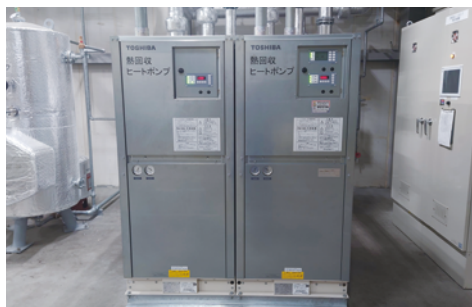
Heat recovery heat pump
