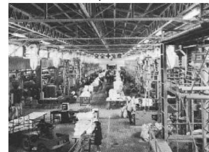
An inside view of the company head office plant
