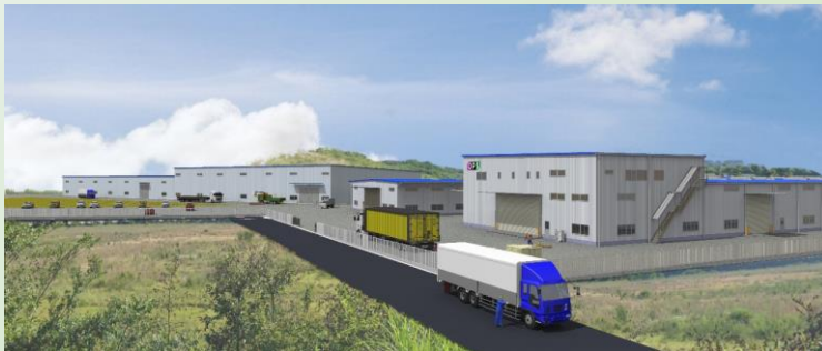
Image of the completed new plant
